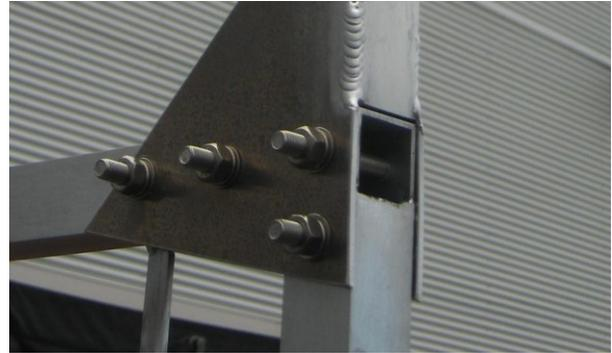
1.4) Install the fasteners from the bags labeled #P2.
