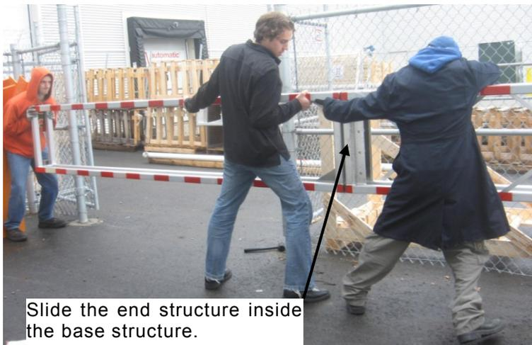
Slide the end structure inside the base structure.
